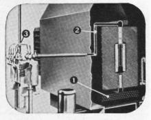
Deseration of condensate not to exceed 0.01 cc. oxygen/liter is available with special Wheeler designs. Note the Deserating Bars (1), the Air-Vapor Suction Line (2), and Tubejet® Ejectors (3).
