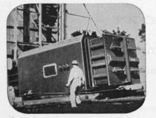
Rectangular Cross Section makes C.H. Wheeler Condensers adaptable to nearly any space or condenser arrangement because the length, width and height of any Wheeler Unit can be varied almost-at will.
