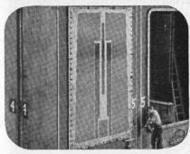
Triple Lane tube layout, another design feature, provides 3 pathways for steam travel, utilizes maximum cooling surface and produces higher condenser vacuums for power generating stations.
