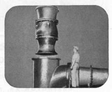
C. H. Wheeler Circulating Pumps, like Condensate Pumps, are easy to inspect and maintain because of "Pull-Out" design. In addition, shafts are heat treated alloy steel and impellers are statically and dynamically balanced for trouble-free operation.
