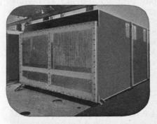
Head Room problems are solved by compact condensers like this one. Turbine floor to basement fleer, in this case, is only 20 ft. The Unit has 65,000 square feet of condensing surface.
