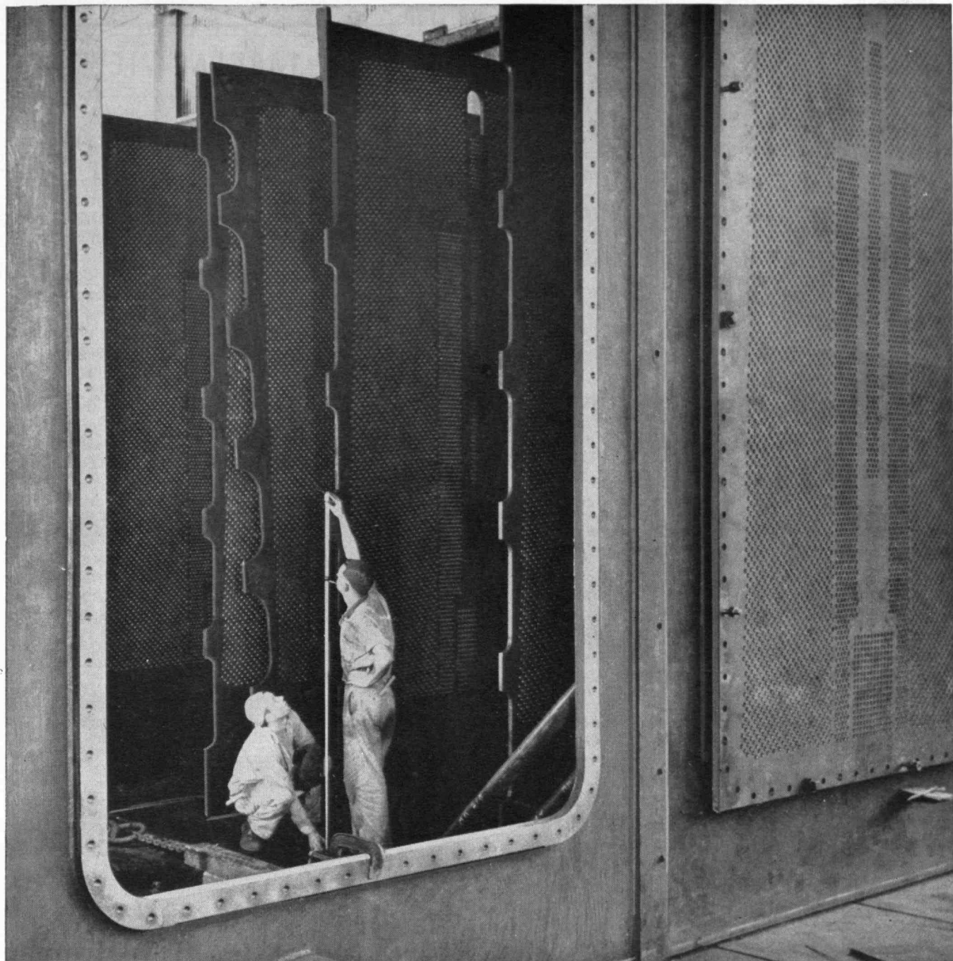
Twin-shell, triple-lane, single-pass Condenser with 187,000 sq. ft. capacity. One of largest units ever built, it was recently installed at large eastern utility.
