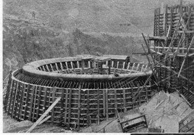
The glory-hole spillway at Owyhee Dam in Oregon is a vertical shaft of the record height of 309 feet, which diverts waste water to a tunnel passing far under the base of the dam and discharging into the river. At the crest the glory hole is 60 feet in diameter. The single ring gate controlling the full circle of the crest is the first of its kind. Above: crest during construction. Right: ring gate in raised position during test.
